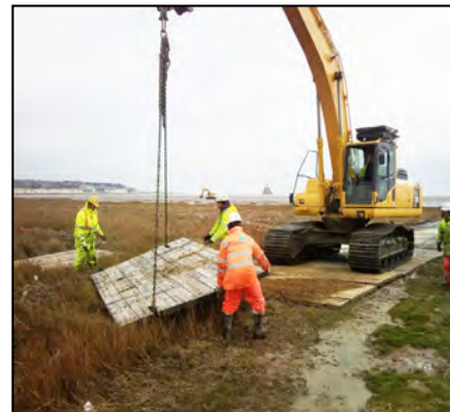
Positioning of Timber Mats
