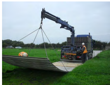
Trackway Installation
